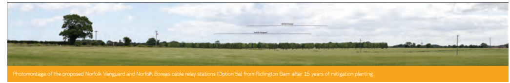
Photomontage of the proposed Norfolk Vanguard and Norfolk Boreas cable relay stations (Option 5a) from Ridington Barn after 15 years of mitigation planting
