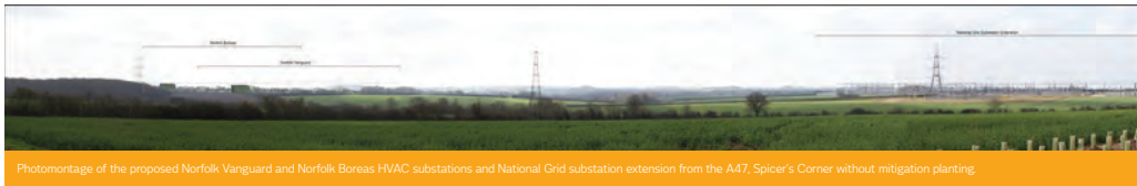
Photomontage of the proposed Norfolk Vanguard and Norfolk Boreas HVAC substations and National Grid substation extension from the A47, Spicer's Corner without mitigation planting.
