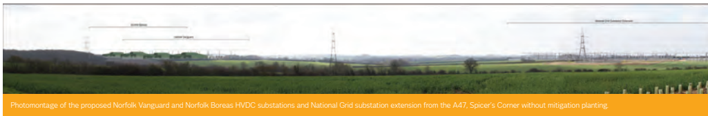
Photomontage of the proposed Norfolk Vanguard and Norfolk Boreas HVDC substations and National Grid substation extension from the A47, Spicer's Corner without mitigation planting.
